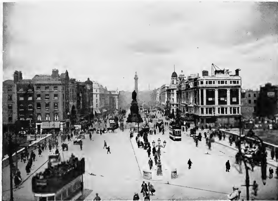
View taken from the south end of O'Connell Bridge, showing the rebuilding as completed in 1921.
