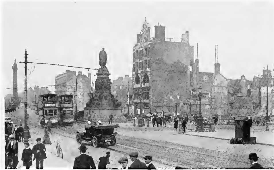
View taken from the north end of O'Connell Bridge, showing the destruction caused in 1916.
