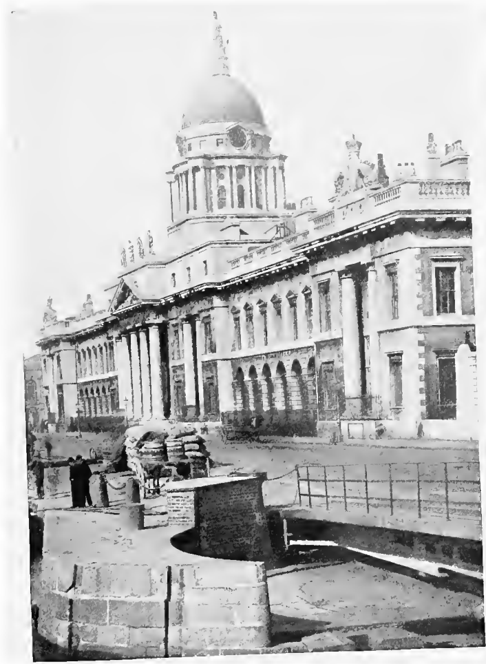
The Custom House before the destruction in 1921
